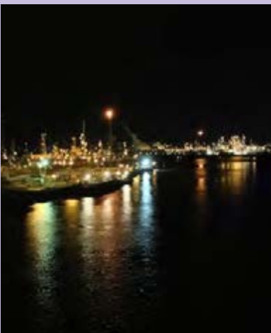
PES facilities at night
