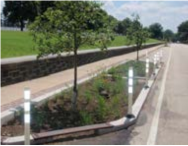
Rainwater garden in curb bump out
