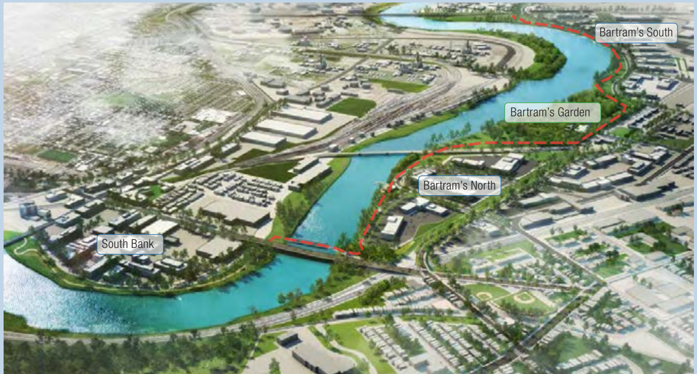
View of the Innovation looking District south with future Schuylkill Banks Trail highlighted in red
