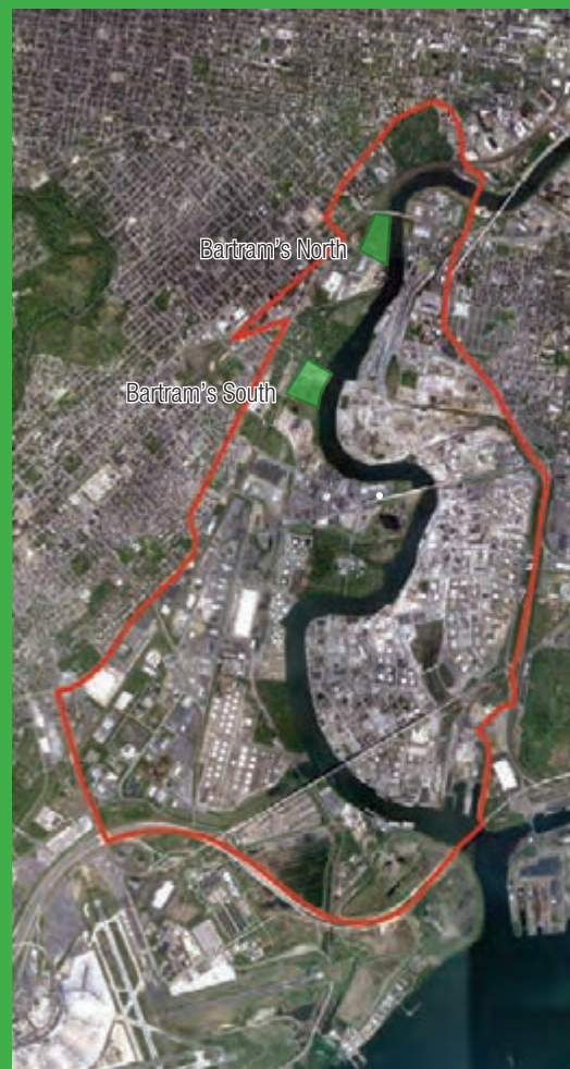
PIDC-owned sites undergoing remediation
